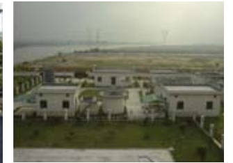
A&E Wastewater Treatment Plant in China
